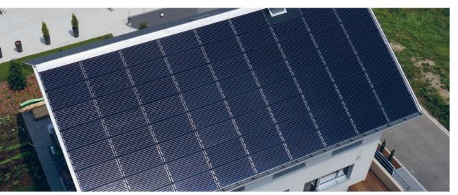
The in-roof system solution – PV generator and roof coverage in one
